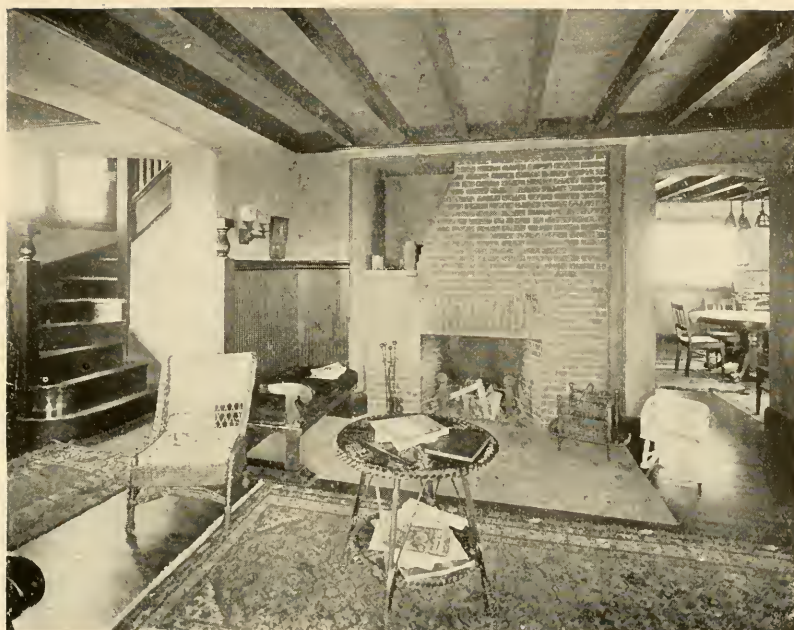
Here the Chimney Breast is Broken Off to Form a Niche
